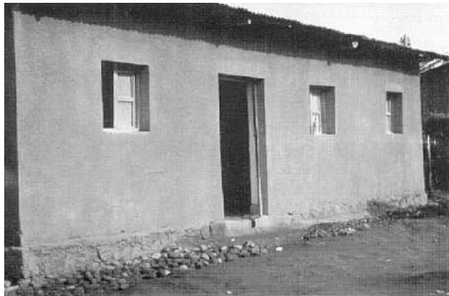
Figure 1: house plastered with lime-pozzolana mix – Rwanda.
