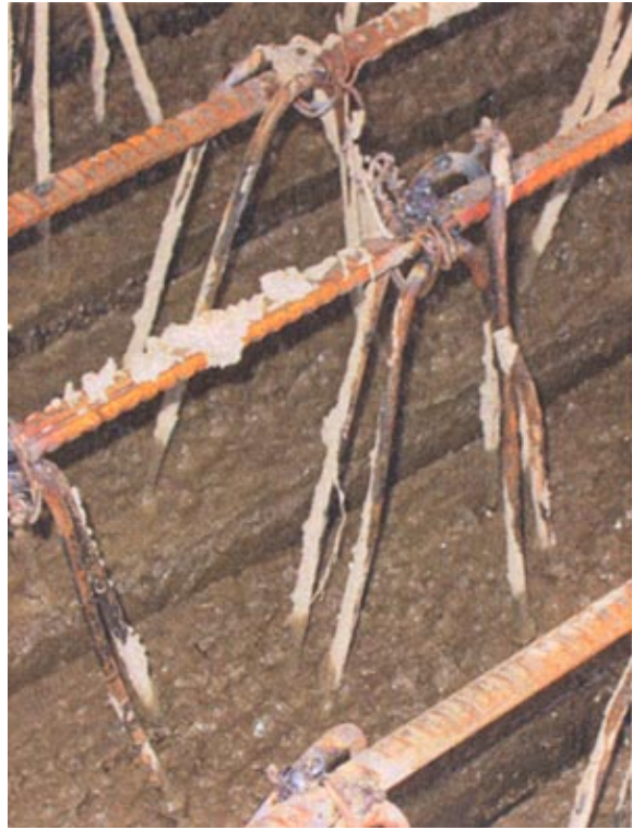
The precast-beams after removing the mould
