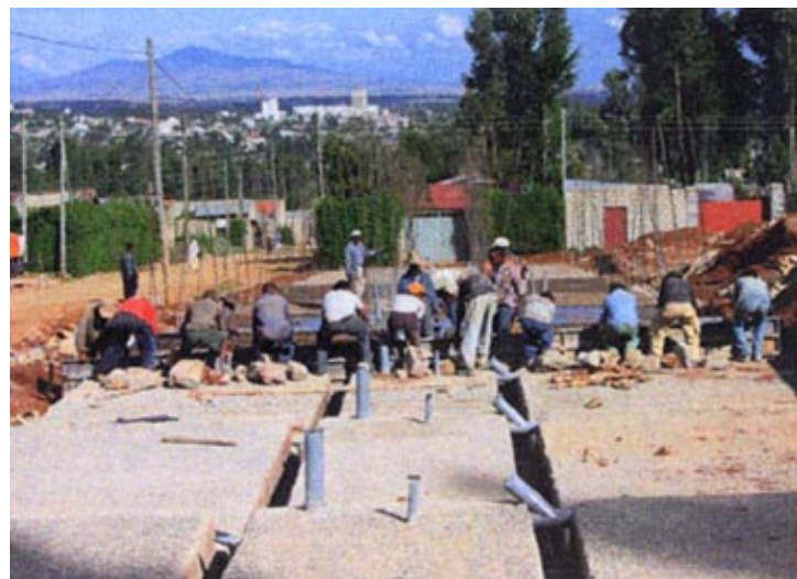
Sanitary pipes are installed
