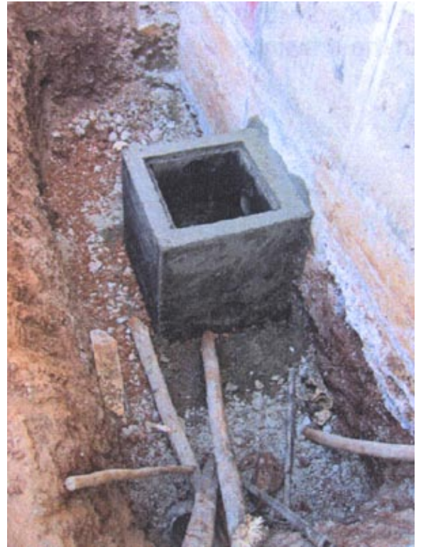
The pit for the manhole
