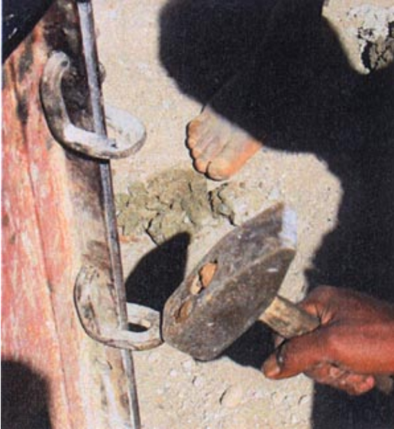
... And locking it by rotating it by 90 degrees
