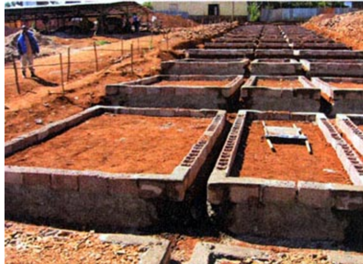
Preparation for combined strip and mat foundation
