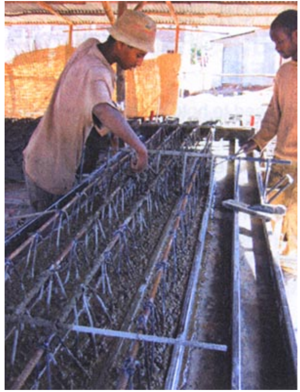
Filling in concrete by hand
