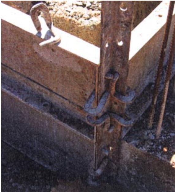
The edge of a formwork-assembly for foundation
