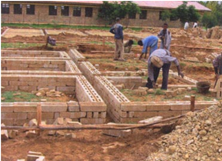
Lost formwork for foundation
