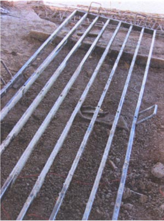
Mould for the pre-cast beams
