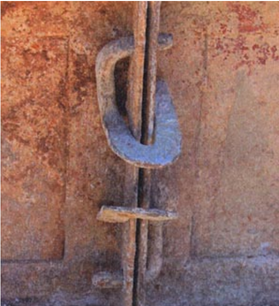
Two clamps mounted on formwork for foundation
