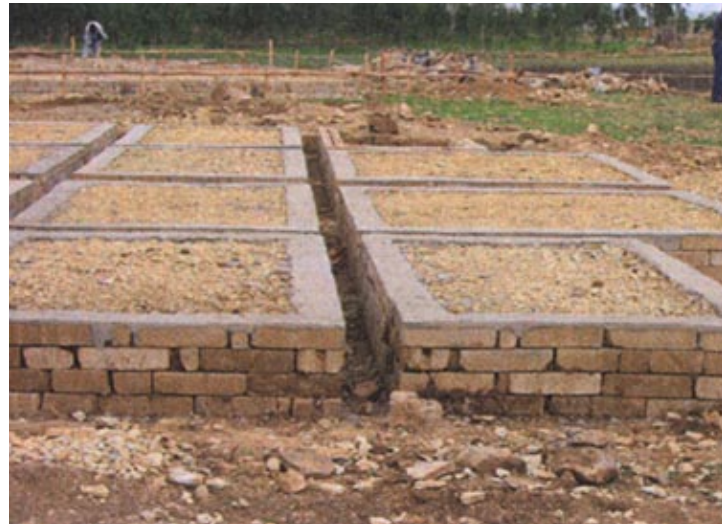
The finished foundation
