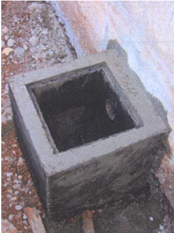
The cast manhole
