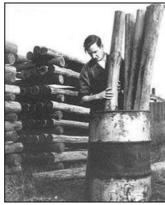
Figure 3. Preservation of timber by dip diffusion
