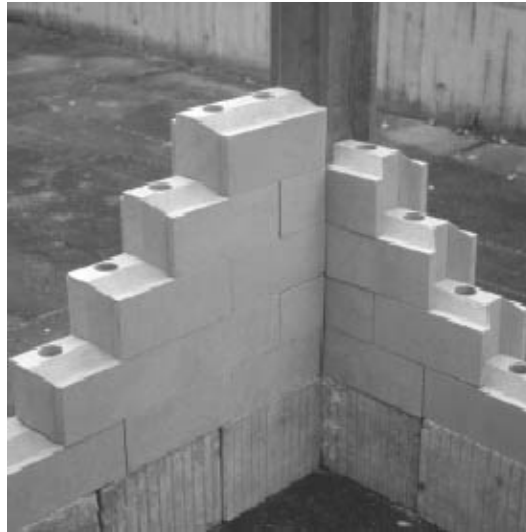
7–15 Improved interlocking system of FEB, Kassel, 2001
