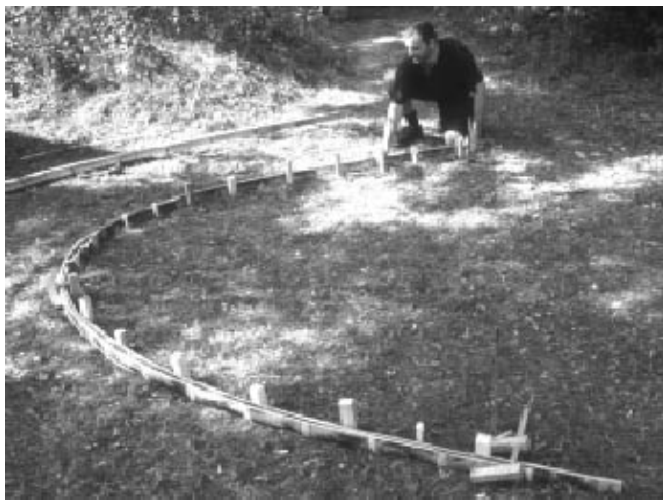
15-7 Construction of the arc with split bamboo
