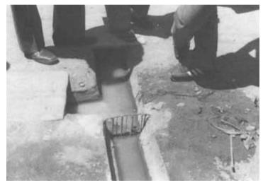
A grille in a small drainage channel. Grilles such as this retain rubbish near the point where it enters the channel, so that the responsibility for cleaning each section can be fairly divided.
